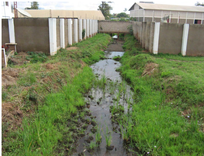
Figure 10. Wetland drained for installation of infrastructure.
