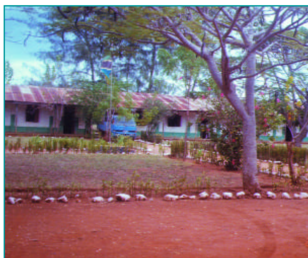
Kilwa Masoko Secondary School.
