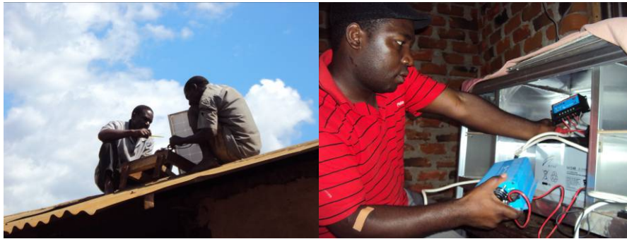
Figure 4. Installation of a solar multi-charger for Mr. Jumanne Hussein in Mihuga village
