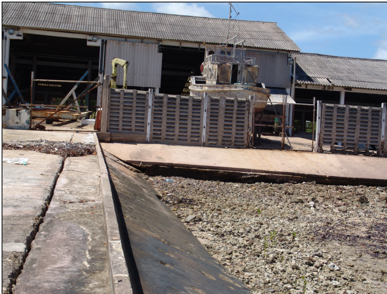
Fig. 13. The jetty in front of the old boatyard at Mbegani, (Top) The eastern (upstream) side of the jetty with no evidence of erosion and (b) the western (downstream) side of the jetty, which was severely affected by coastal erosion
