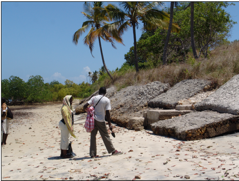
Fig. 13: Gabion seawalls used to protect an eroding Holocene beach ridge located about 2 km from Mbegani.
