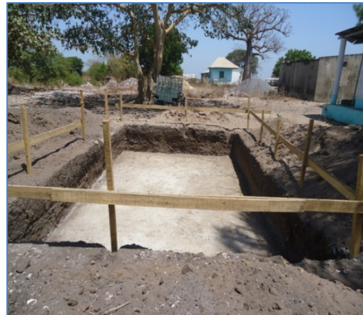
Jeshwang sanitation facilities construction
