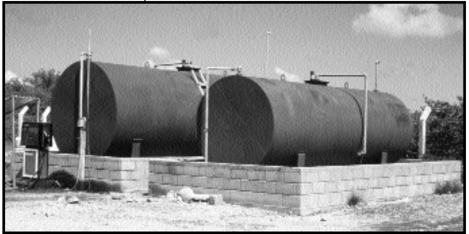
Fuel tanks and other containers with hazardous materials should be surrounded by retaining walls in case of spills.
