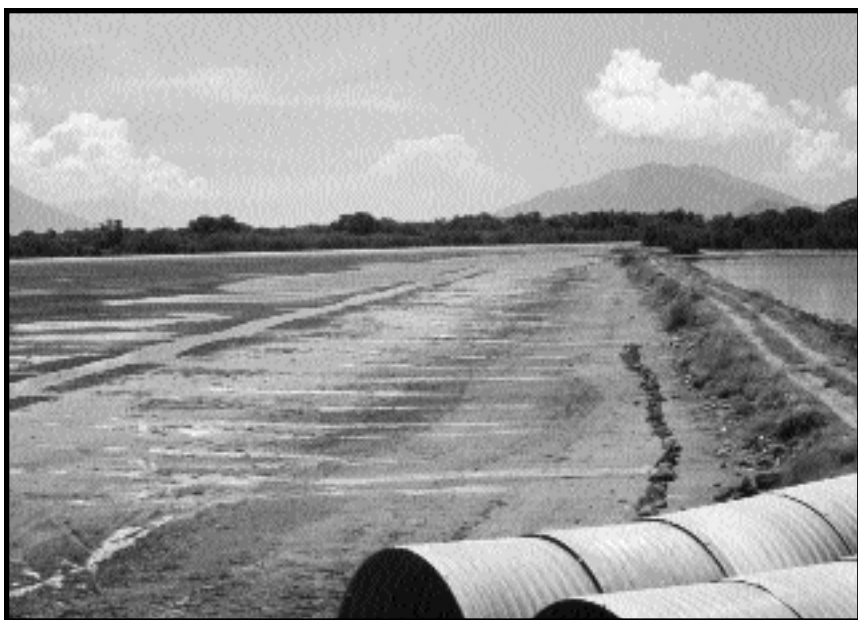
When properly applied, lime should cover the bottom of the pond. An inadequate amount has been applied to the pond above.
