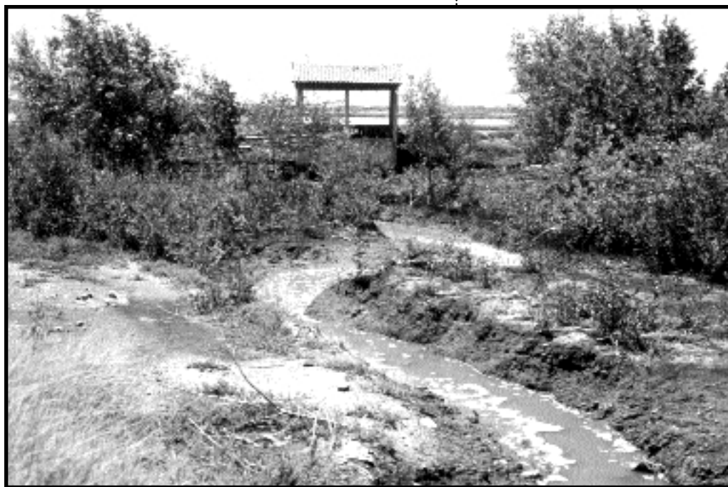
The pumping station is situated where water volume is low and may be of poor quality.
