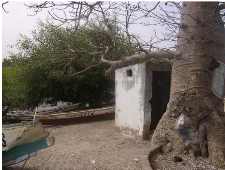
Figure 6. Pit latrine at the Lamin Lodge site located within 10 meters of mean high tide elevation.
