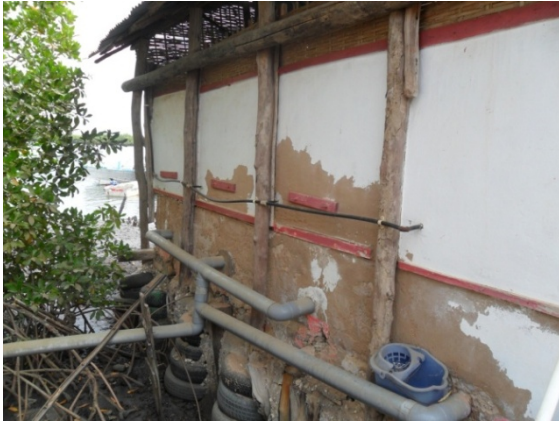
Figure 4.7 (a): Drain pipes from Lamin Lodge toilets emptying directly into the estuary
