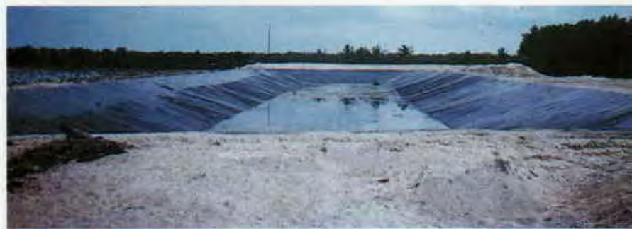
Laem Talumpuk community's reservoir.
