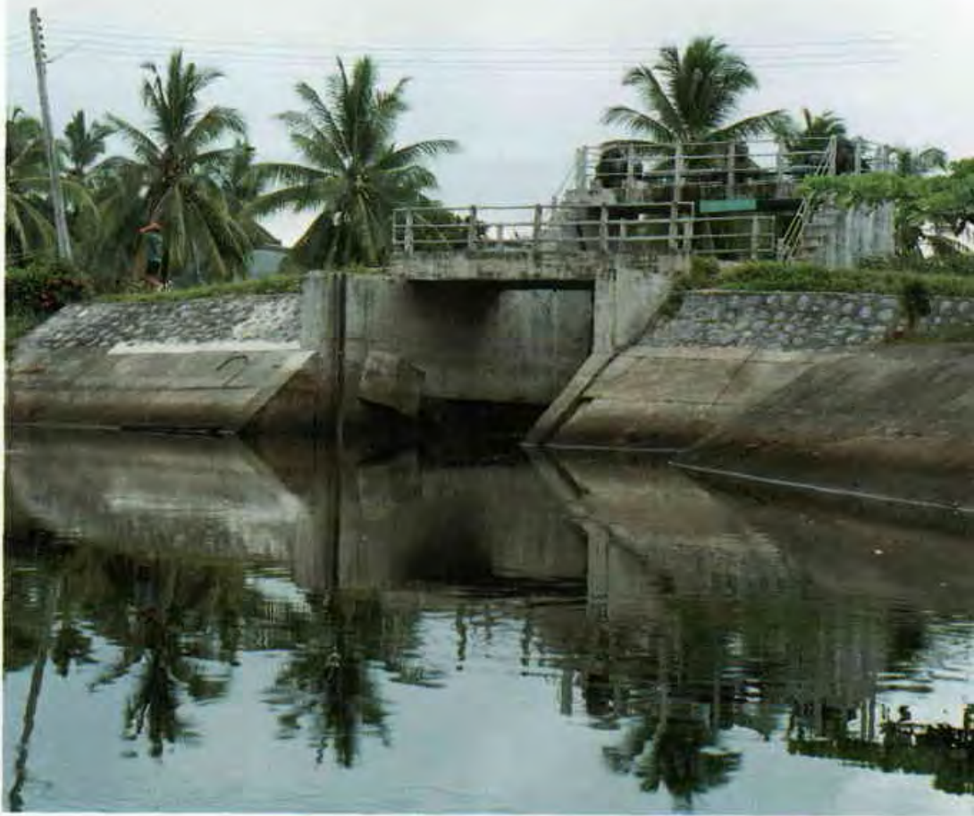
Khlong Bang Chak water gate.
