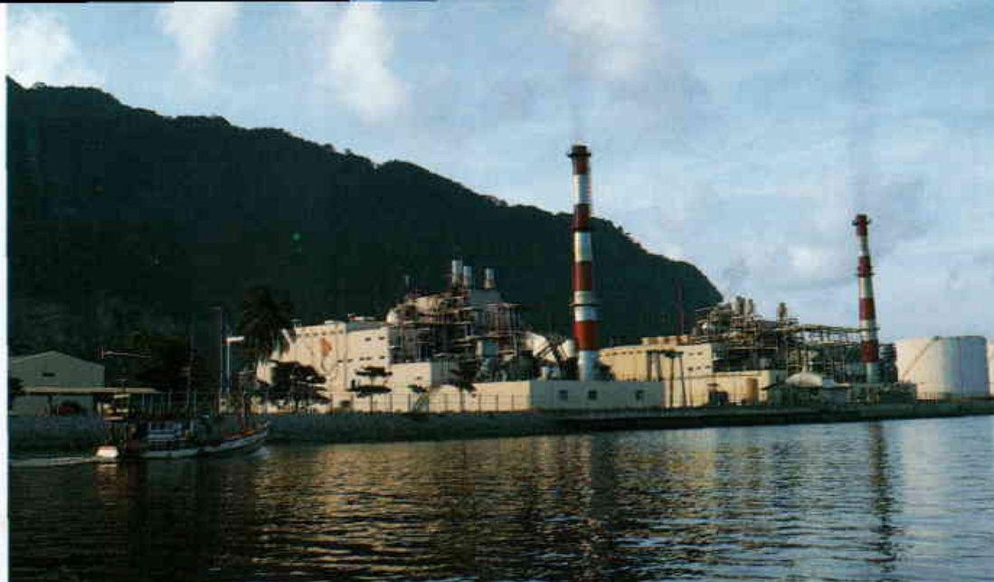
Power generating plant at Nakhon Si Thammarat.
