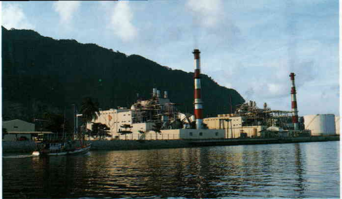
Power generating plant at Nakhon Si Thammarat.
