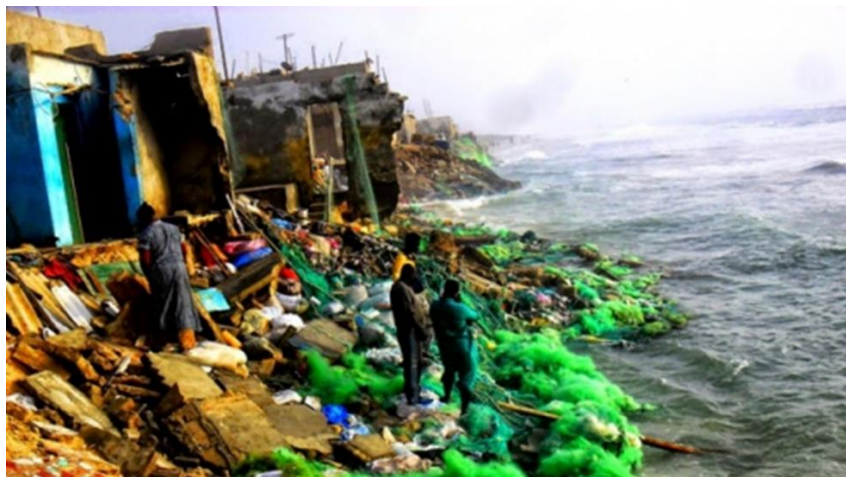
Figure 4. Houses destroyed by flood in Saint Louis
