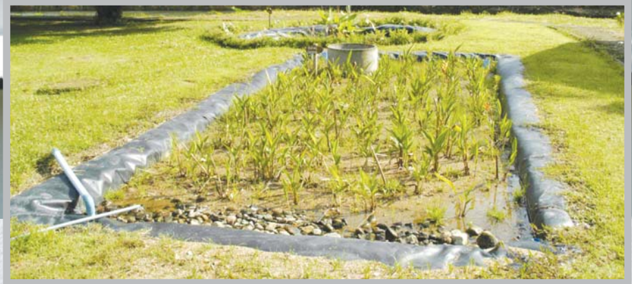
Constructed wetland for wastewater management
