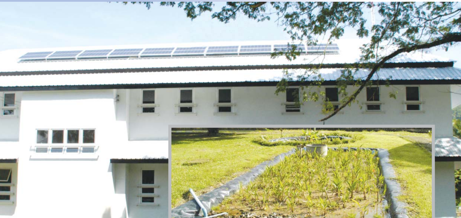
Energy efficient rooftop solar panels
