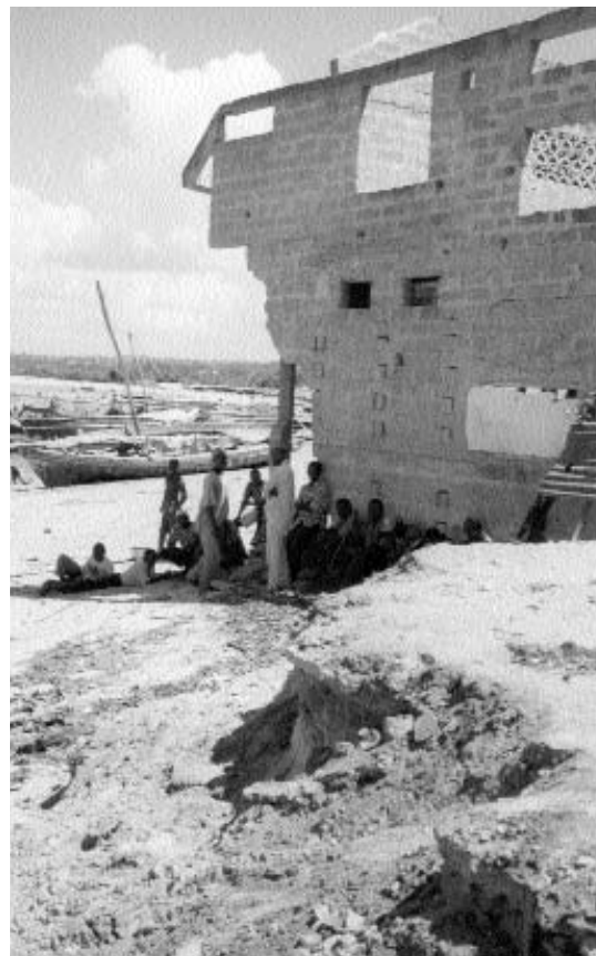
Coastal erosion in Tanzania
