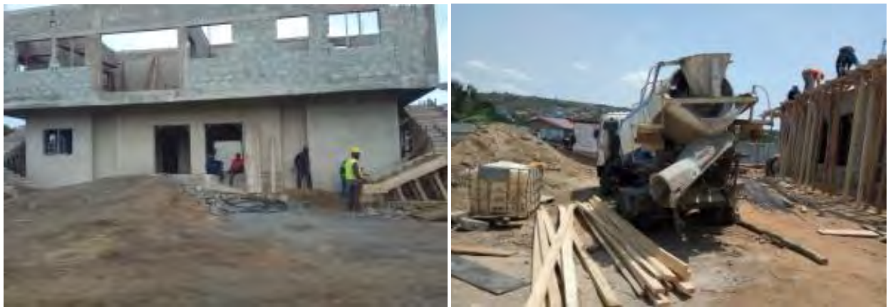
Figure 20: DAA Fisheries Training Center under Construction
