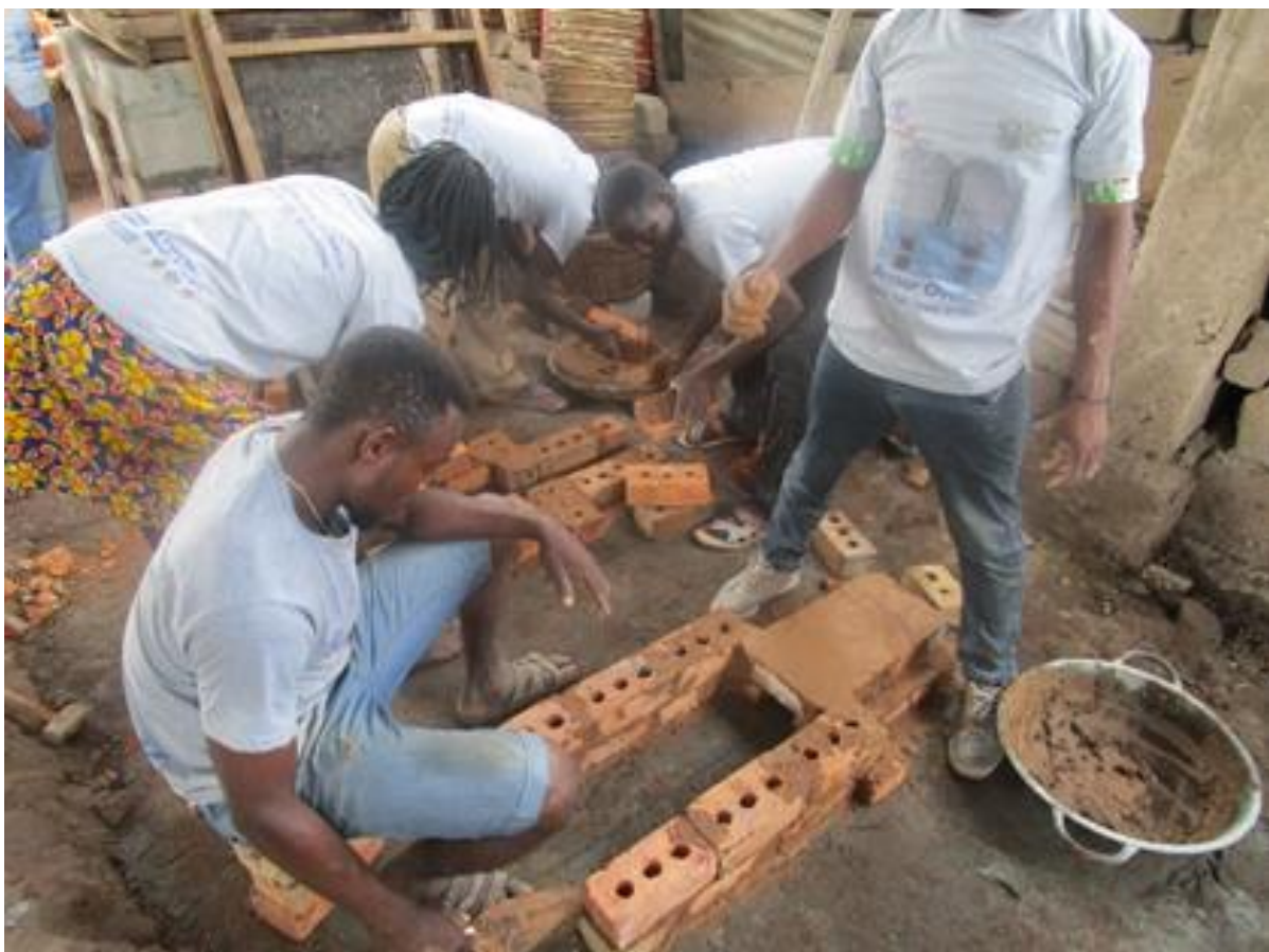
Figure 6. Both genders being trained on how to construct the Ahotor oven
