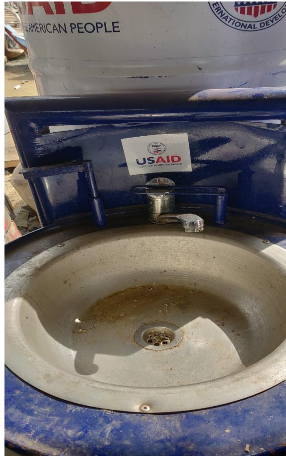
Figure 14 Broken down Handwashing station at Awudin
