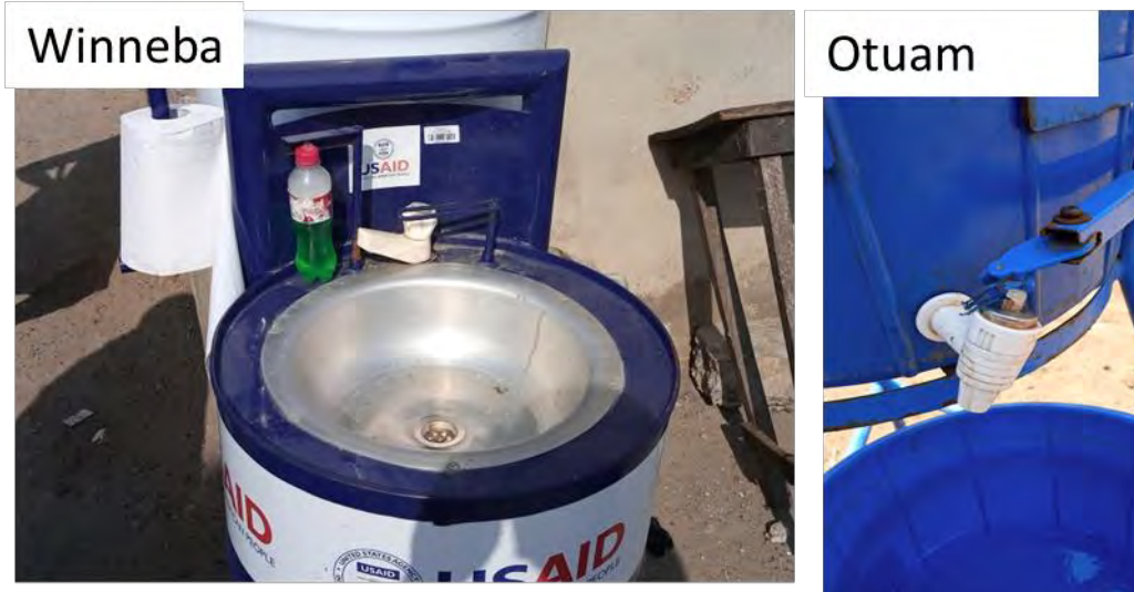
Figure 8 Broken taps replaced with improvised taps
