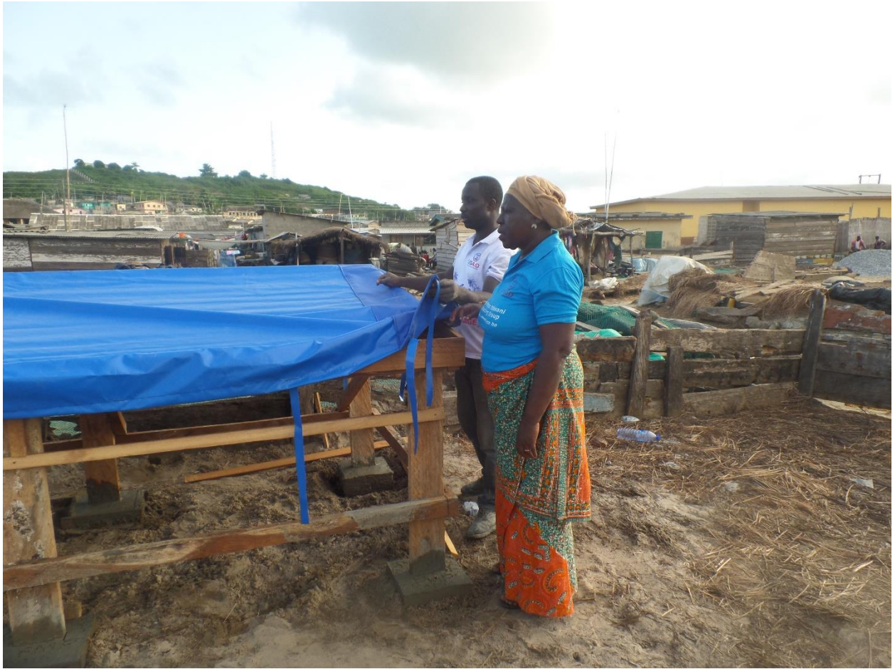
Figure 7: Mr. Abraham Asare and Mrs. Lydia Sasu of DAA inspecting the finished raised racks before handing over to the beneficiaries
