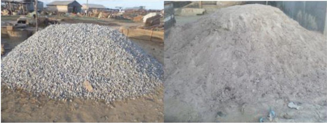
Figure 4: Some materials used in securing the footing of the racks during the construction process
