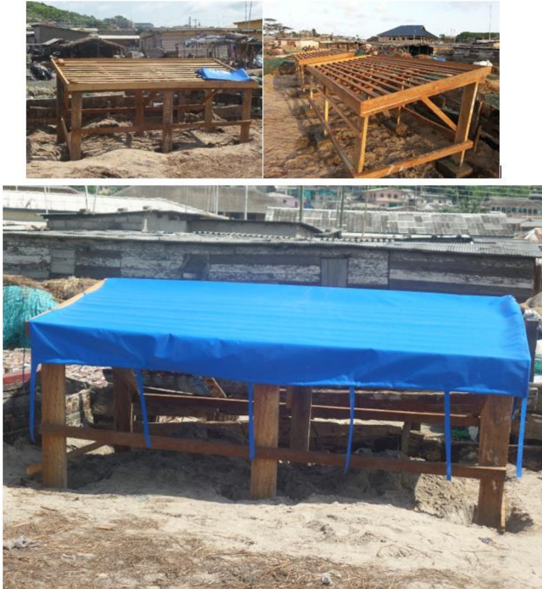
Figure 6: Finished raised drying racks in Apam with a tapoline cover
