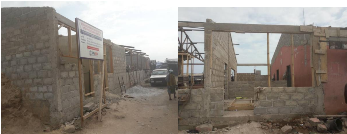
Figure 6 Outside Structure on September 9, 2017
