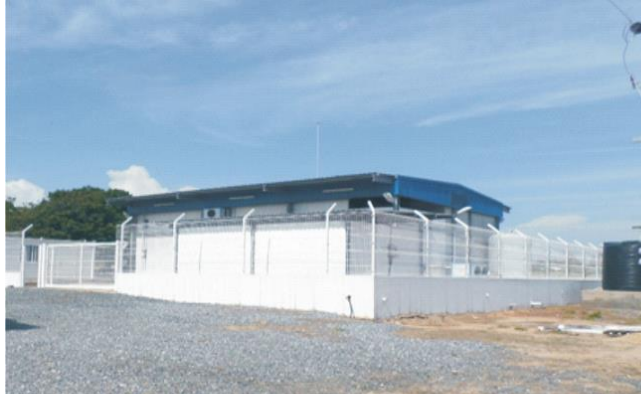
Figure 101. Cold store facility
