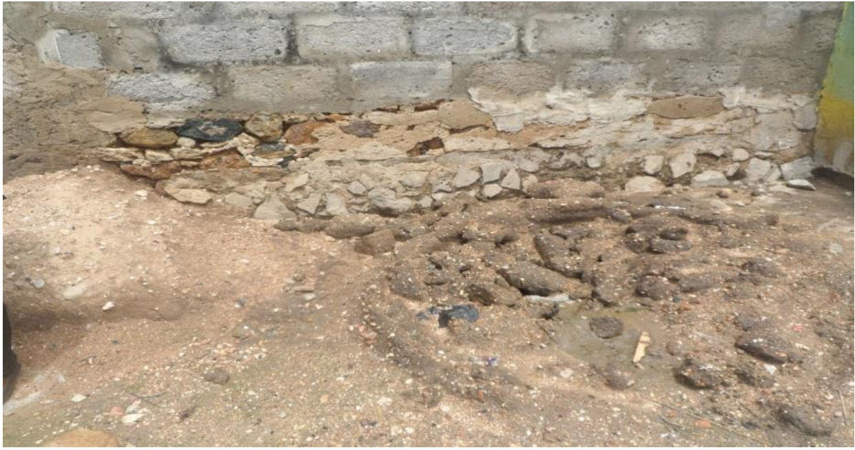
Plate 8 Bad Oven (totally collapsed in Winneba community)
