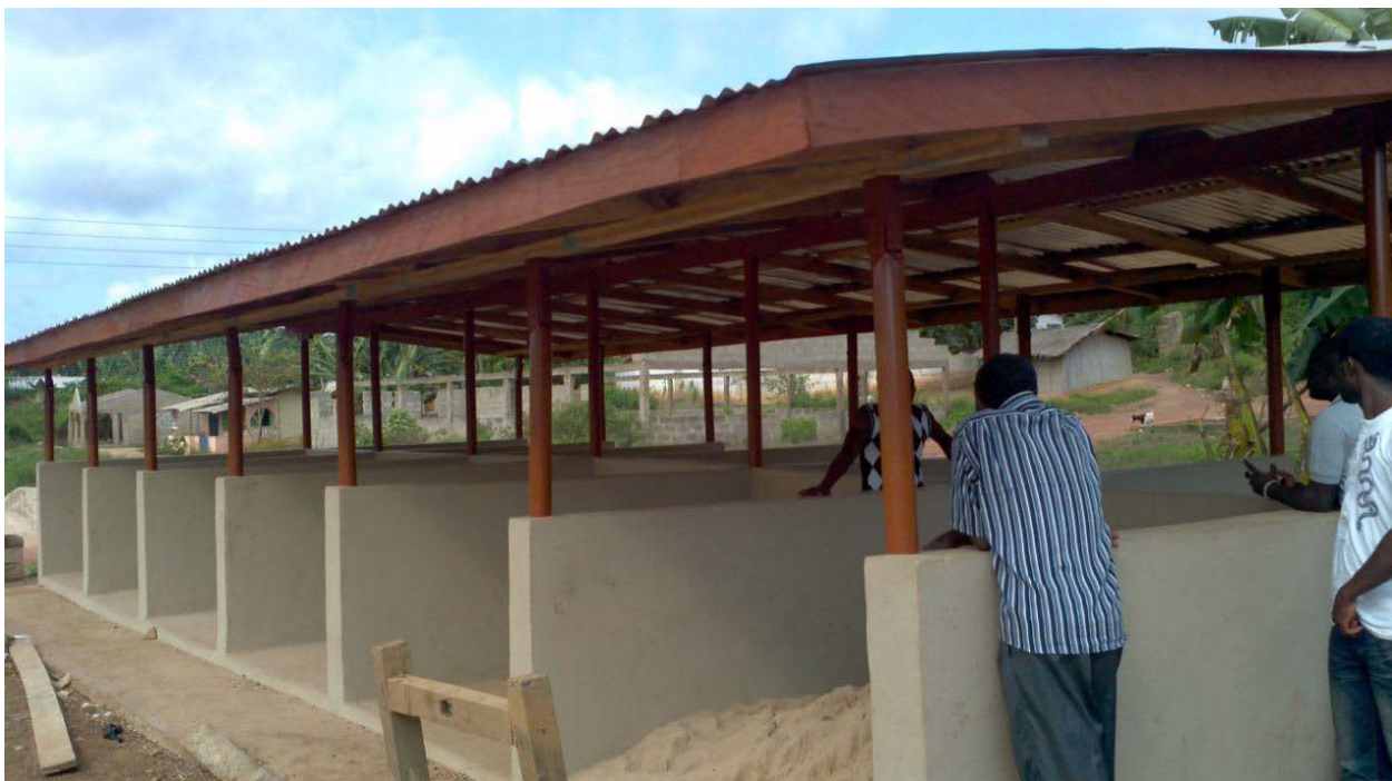
Figure 14: A near complete Akwidaa Market donated by USAID and the ICFG Initiative
