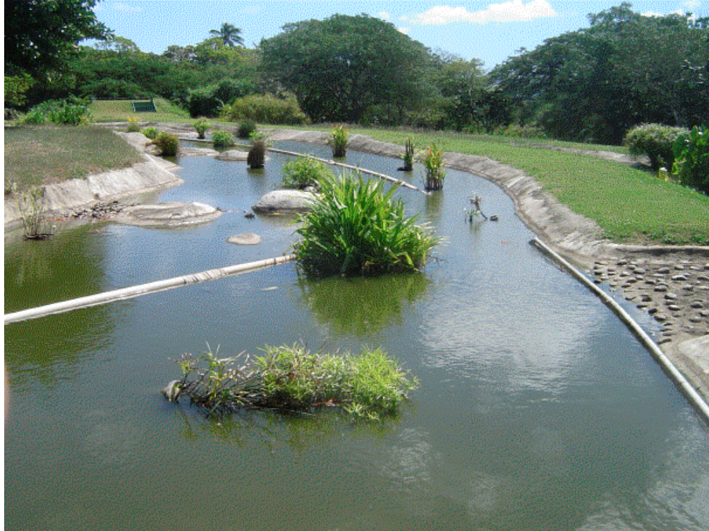
Figure 14: One of a series of three surface-flow constructed wetlands set up to receive treated wastewaters recirculated from the adjacent irrigation water storage pond. (Photo: Chris Tanner).
