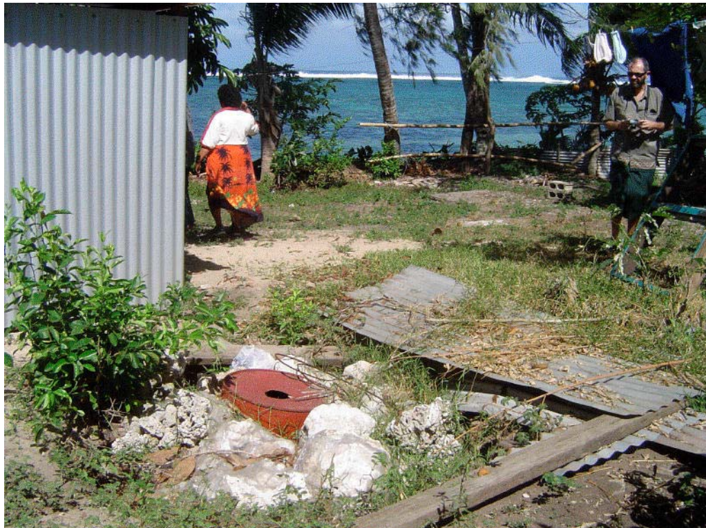
Figure 9: Recently constructed, low-cost village household soakage pit awaiting connection to flush toilet system. The soakage pit comprises two perforated 200L steel drums set one above the other in a large hole, surrounded by coarse coral rock. The base of upper drum and top of lower drum are removed to create a single chamber. (Photo: Chris Tanner).
