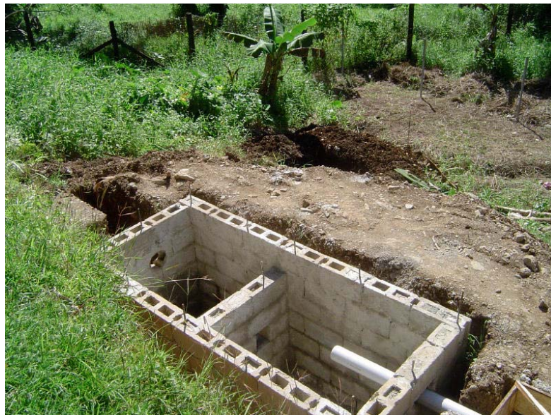
Figure 5: Demonstration two-chamber septic tank being constructed at the Fiji School of Medicine Environmental Health School in Suva (May 2004). One of the key issues with on-site fabrication of septic tanks is achieving a watertight chamber, so as to
