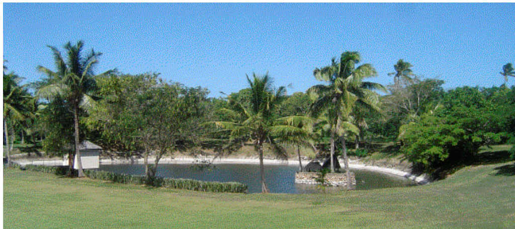
Figure 13: One of two treated wastewater irrigation storage ponds at the Fijian Hotel. The treated wastewater is used to irrigate the hotel golf course. (Photo: Chris Tanner).
