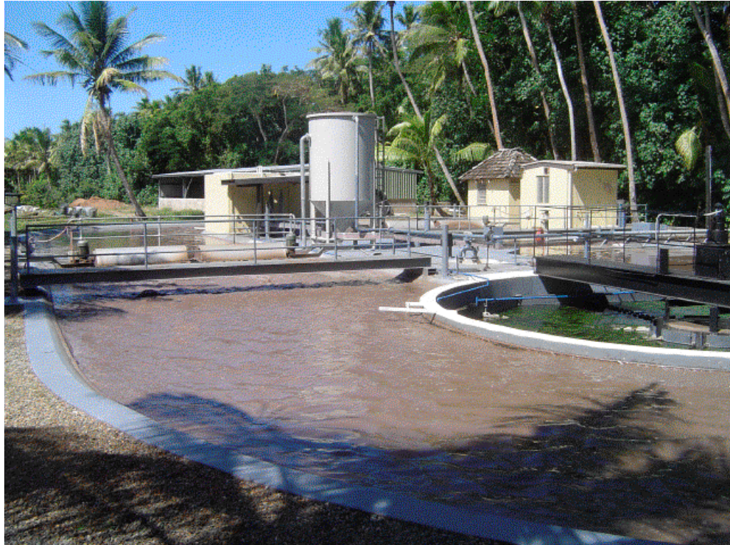
Figure 12: Recirculating oxidation ditch activated sludge wastewater treatment system in operation at the Fijian Hotel. (Photo: Chris Tanner).
