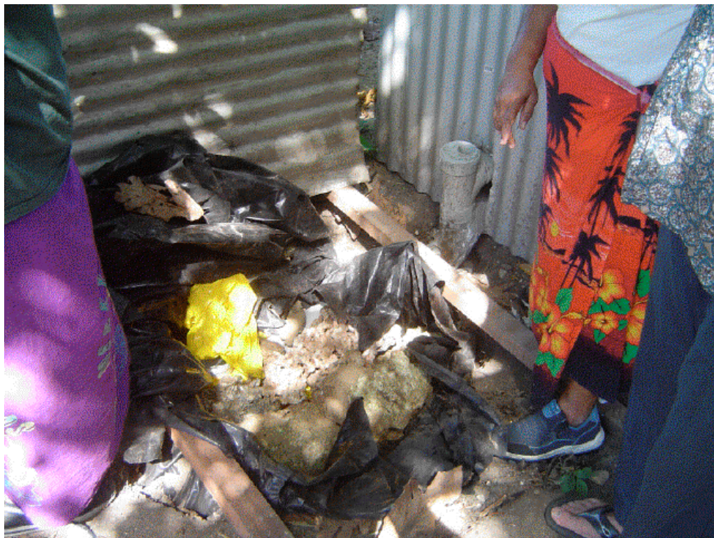
Figure 10: Recently connected village household soakage pit for toilet waste disposal. The still incomplete system has been partially uncovered to show the construction method used. Coarse coral rock is visible surrounding the central perforated steel drum. Note the close proximity to the toilet building. (Photo: Chris Tanner).
