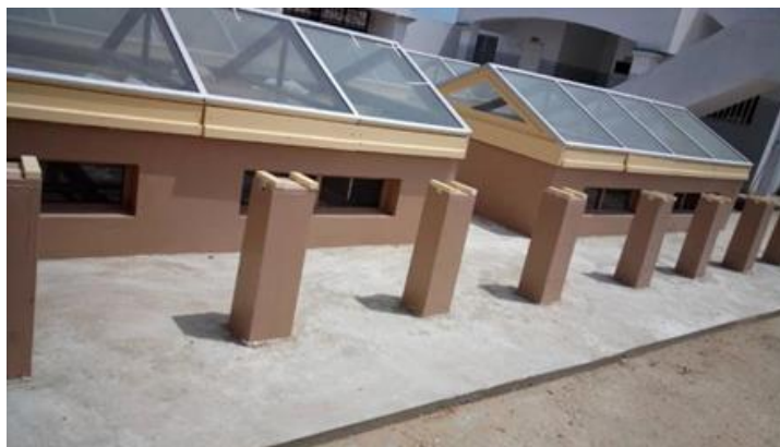
Figure 21. Solar dryers installed at the Cayar modern processing center
