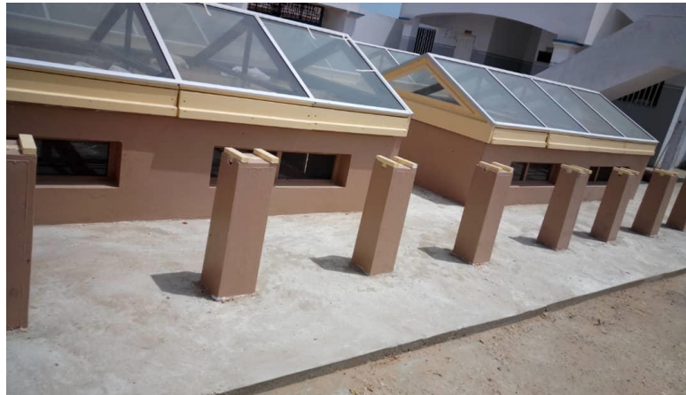
Figure 27. Solar dryers installed at the Cayar modern processing center
