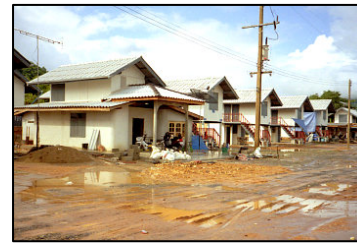
Figure 10. Standing water after a rain storm in Village 7.
