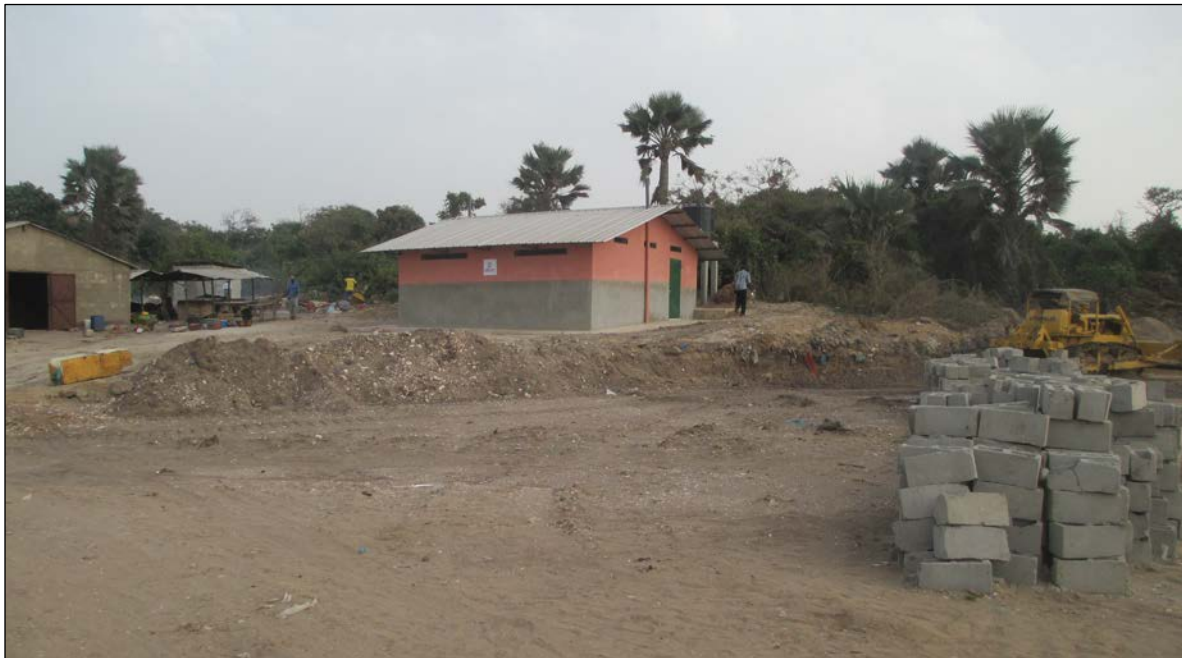
Figure 15. (From top left). Georgette Yarboi-Quayson of USAID/West Africa outside the Brufut fish landing site WASH facility. Interior views. (Bottom) One of the two toilet blocks at Brufut.
