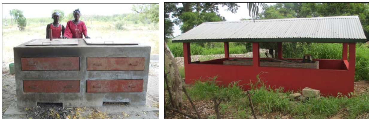
Figure 20. (left) Pilot oyster smoking oven technology transferred from Senegal, constructed at Kamalo oyster site. (right) Improved design oyster smoking infrastructure scaled up to 15 harvesting sites with UNDP funding.
