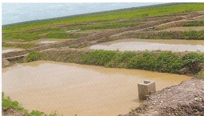
Fig. 4. Tilapia pond at Sapu showing monk drain at deepest end of the pond and the emergency spillway at the shallow end of the ponds spilling into a shallow drainage canal. Photo by Famara Darboe.
