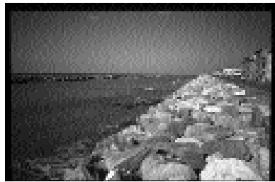
Figure 2. Seawall and breakwaters.
