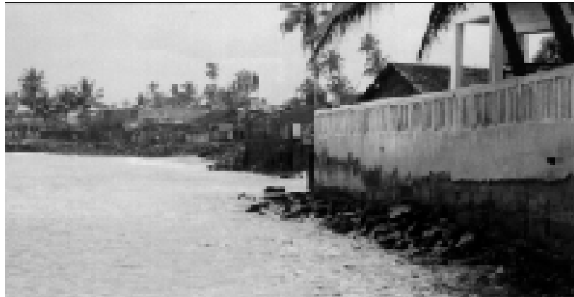
Coastal erosion is a major threat to poorly planned development in Hikkaduwa
