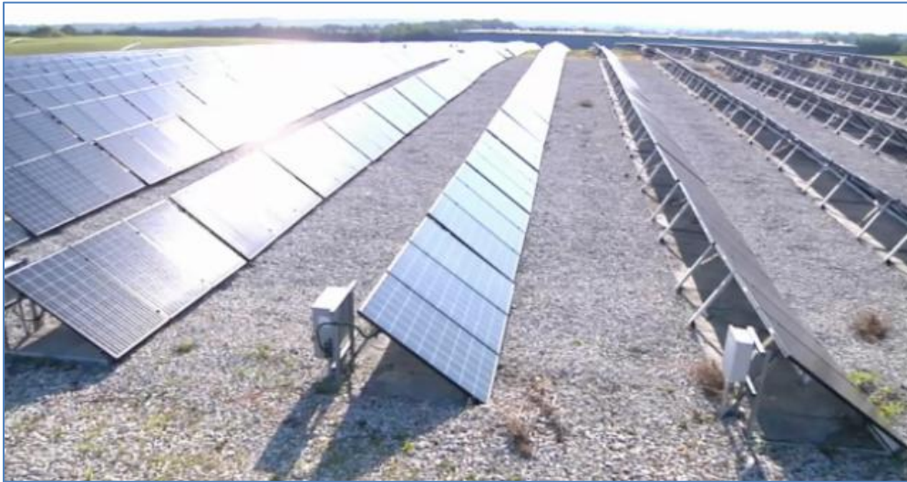
Ch. 2 Figure 3. Rigid Crystalline Photovoltaic Panels in a Fixed Tilt Array (PPL 2010).
