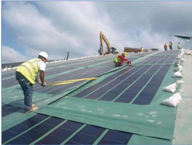
Ch. 2 Figure 10. Geomembrane Cap with Incorporated Solar Panels on Landfill Side Slopes in New York State (Barton and Loguidice, P.C. 2011).
