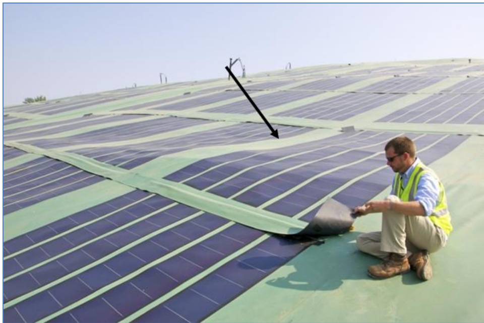
Ch. 2 Figure 7. Flexible Solar PV panels with Arrow Indicating Slope Change (Adapted from CES 2011(a)).
