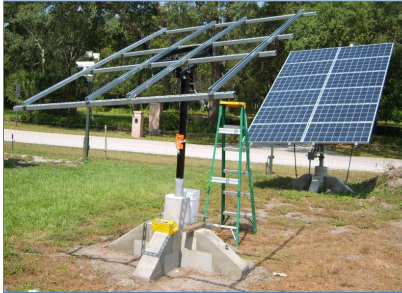
Ch. 2 Figure 4. Mount and Racking for Dual Axis Tracking Rigid Crystalline PV Panel (Parish 2009).
