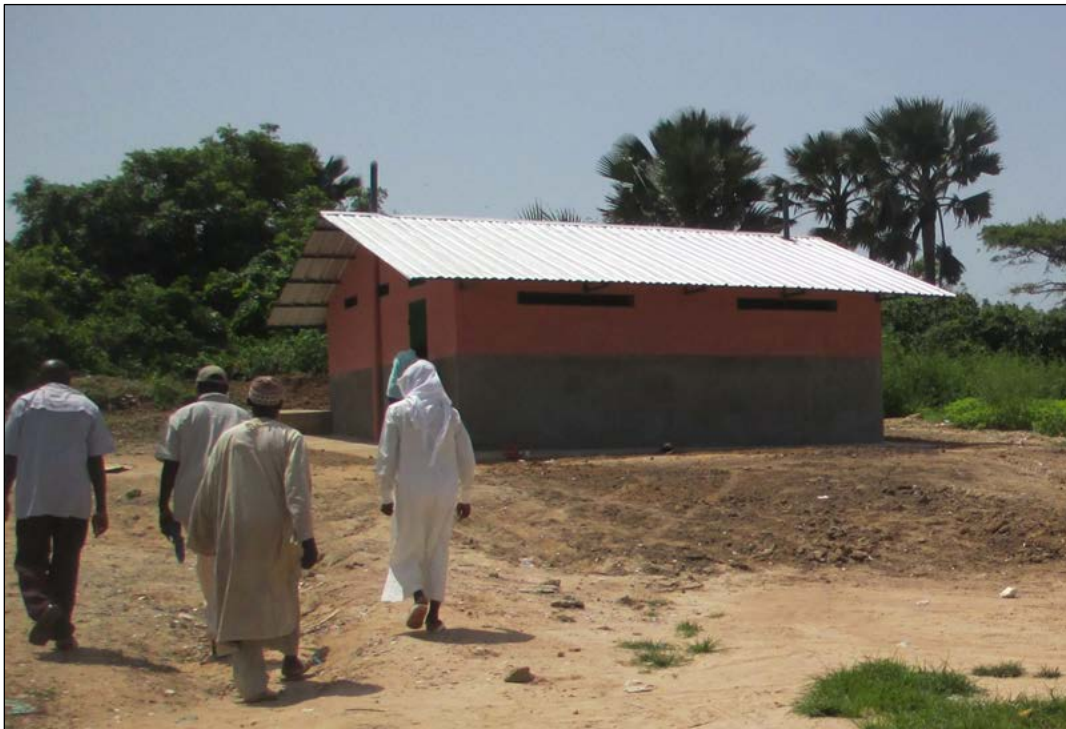
Figure 25. New WASH facilities at Brufut fisheries landing site.
