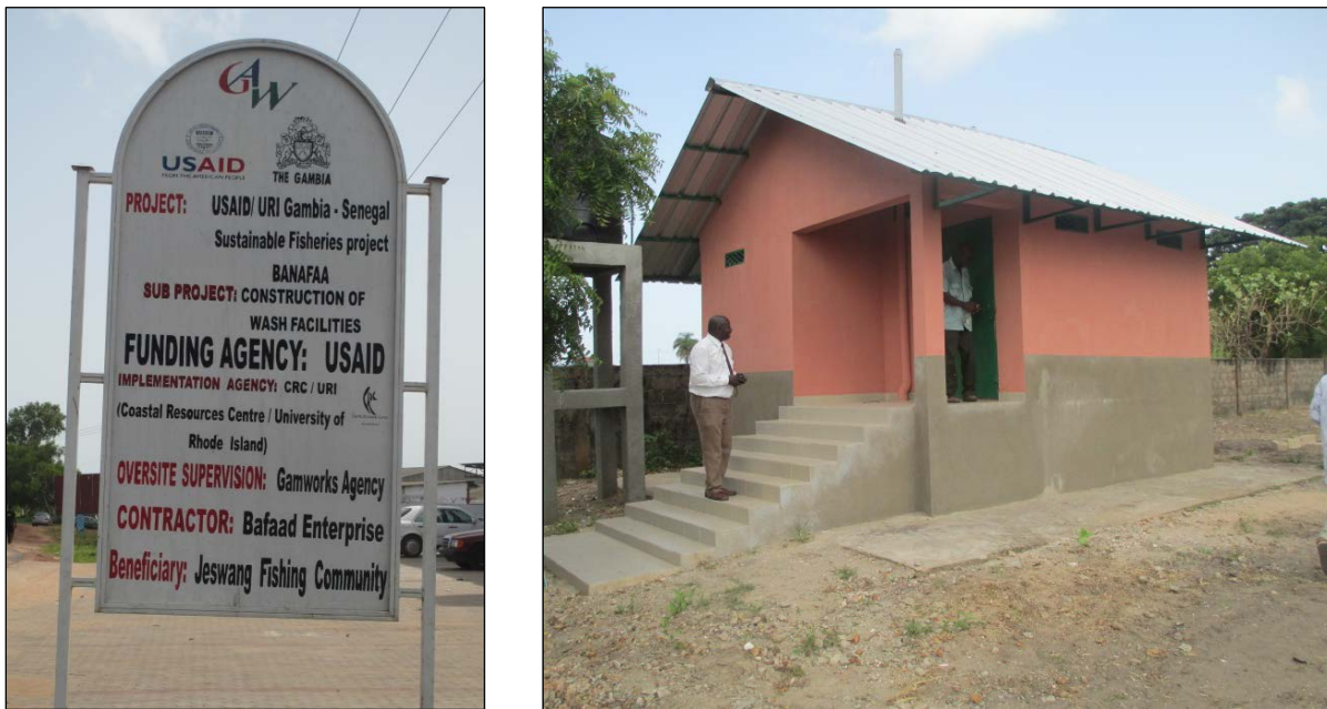
Figure 23. Old Jeshwang fishing site WASH facilities and signage.
