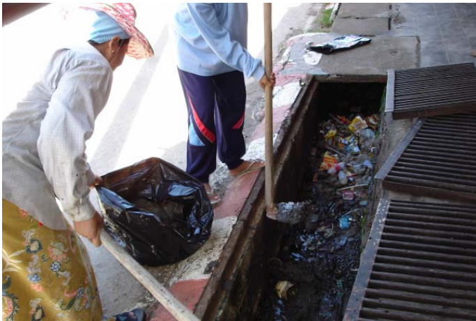
Tsunami survivors in a village in Suk Sumran Sub-District, Ranong Province, Thailand, clean out the village's sewer line with the help of USAID's Cash for Work program.
