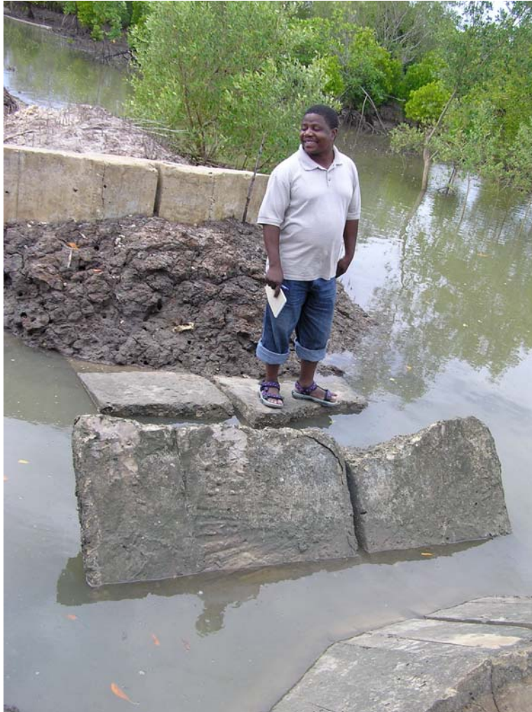
Extension Agent Mr. Muganga stands on the ruined main water supply gate of the Kirago Farm caused by high spring tides overflowing the main perimeter dike
