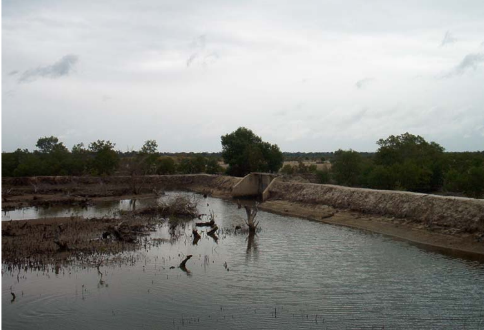
Main water gate at Regent Enterprises salt pans in Bagamoyo
