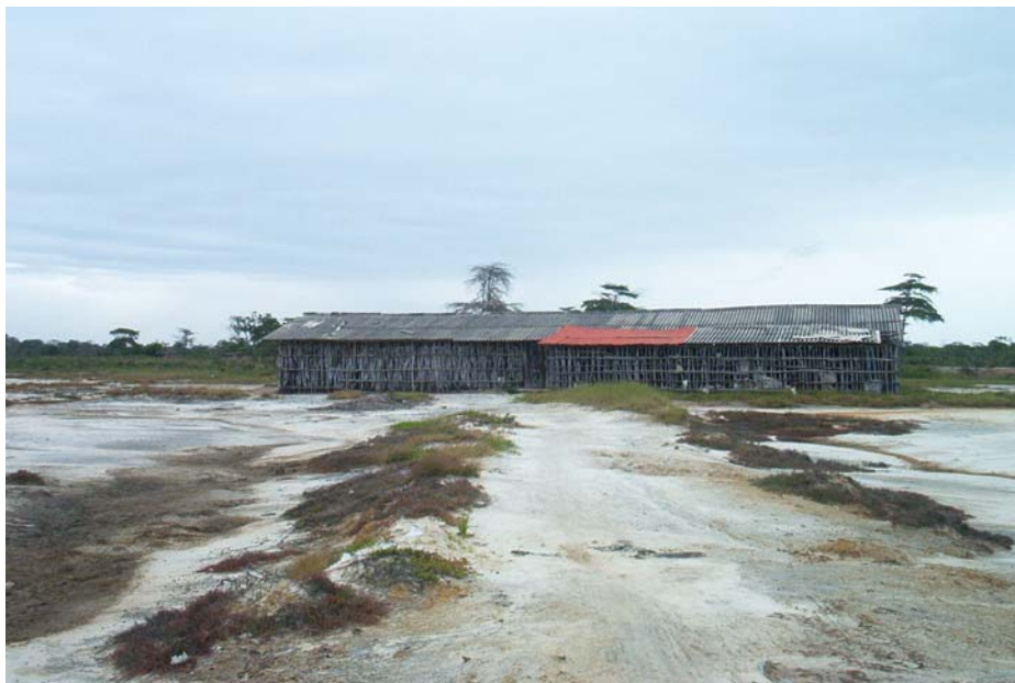
Salt storage warehouse at the Regent Enterprises salt pans
