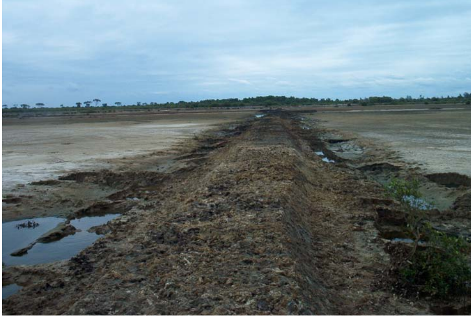
Newly constructed dike at Regent Enterprises site using quality clay-loam blocks and proper slope, base and crown dimensions
