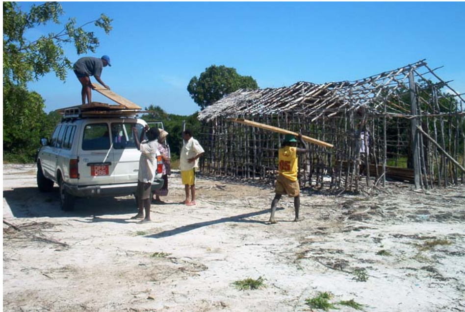
Moving lumber for wooden gate construction to Mukadam Farm
