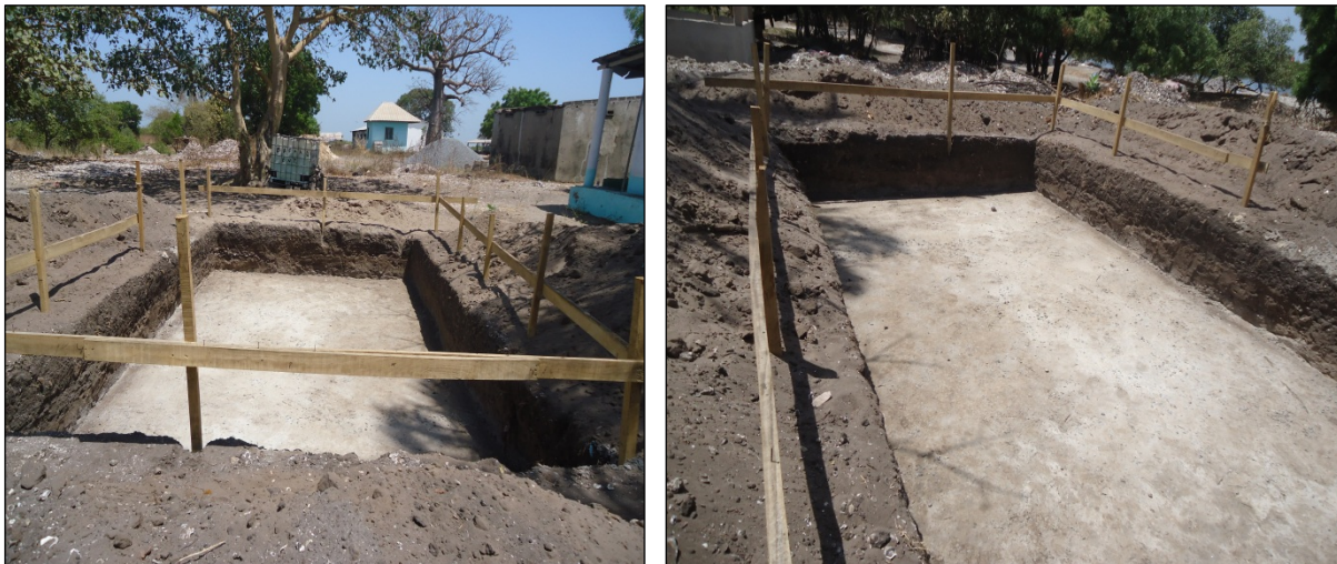
Figure 29. Jeswang Oyster Landing and Processing Site, Excavation Complete and oversite concrete cast
