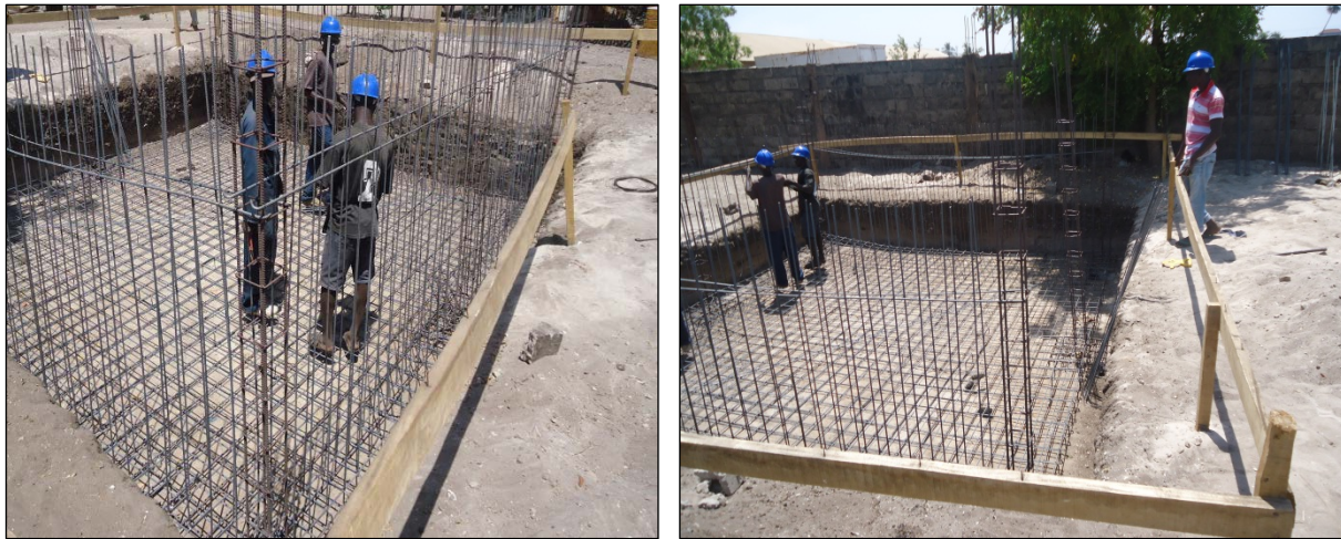
Figure 28. Jeswang Fish Landing Site, concrete is done and reinforcement is being fixed for tank
