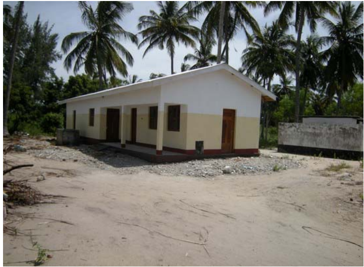
Newly constructed dispensary in the Mkwaja village
