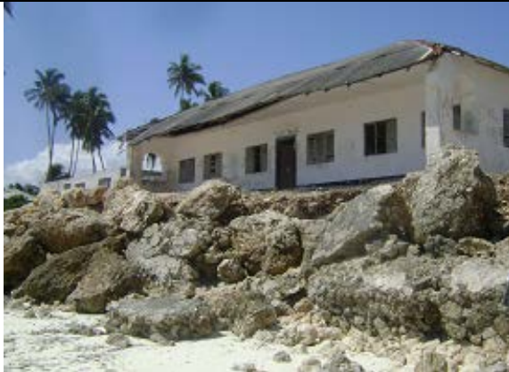
Large stones from a fallen wall at Jambiani
