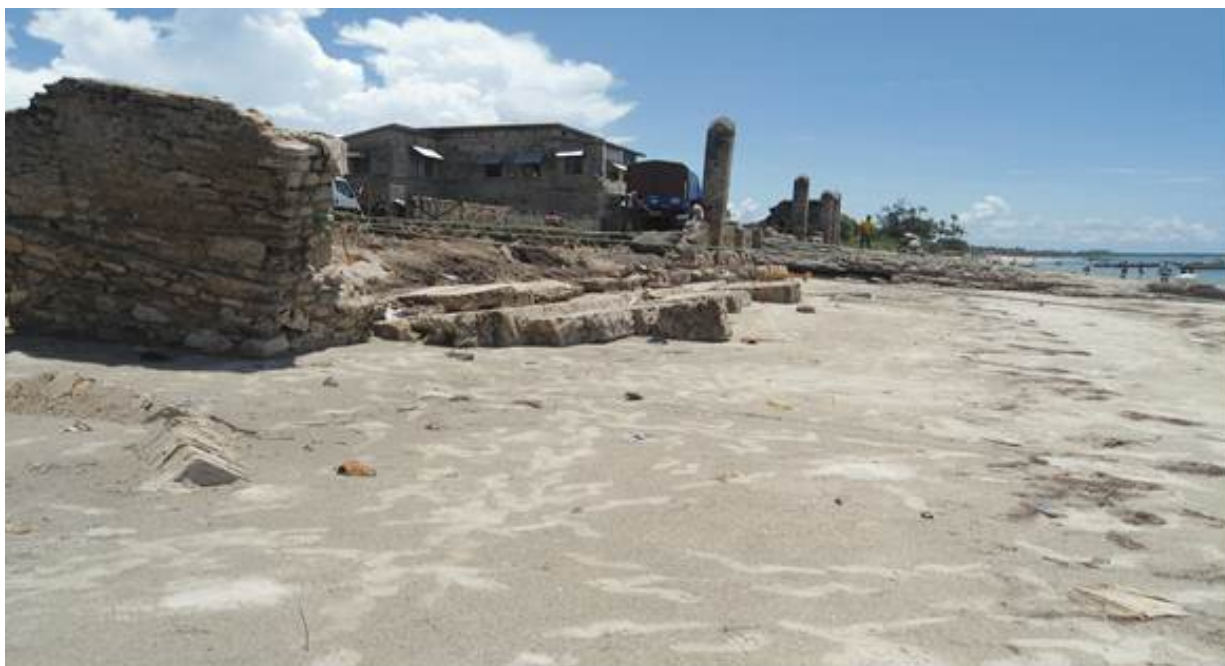
Figure 7 Beach erosion collapsing old Boma important tourist visit areas at “Kastamu/Customs”, Bagamoyo
