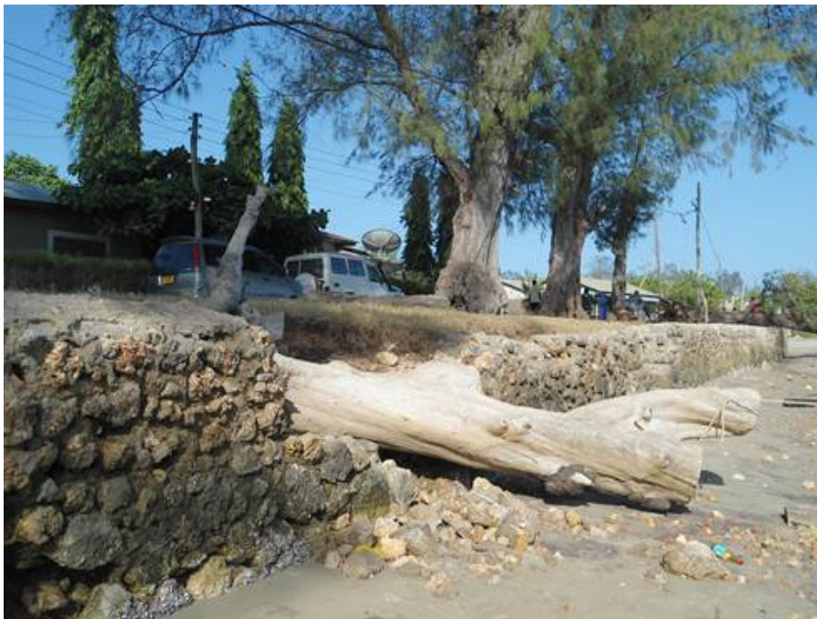
Figure 8. Photo of Pangani river wall near UZIKWASA Office, March 2012
