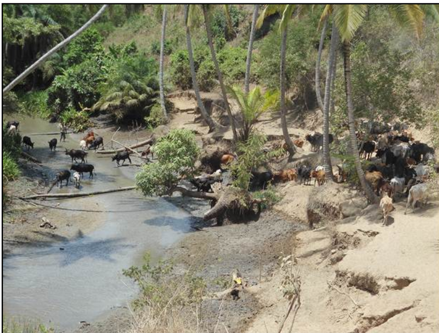
Figure 6. A freshwater stream at Kigurusimba village with serious erosion as a result of cattle trampling
