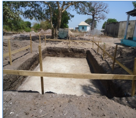
Jeshwang sanitation facilities construction
