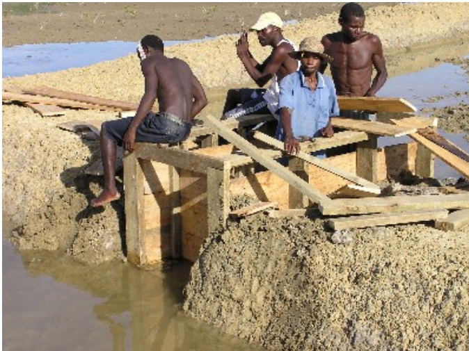
Construction of a secondary gate in Mkadam site in Tanzania with the assistance of former volunteer Edwin Requintina
