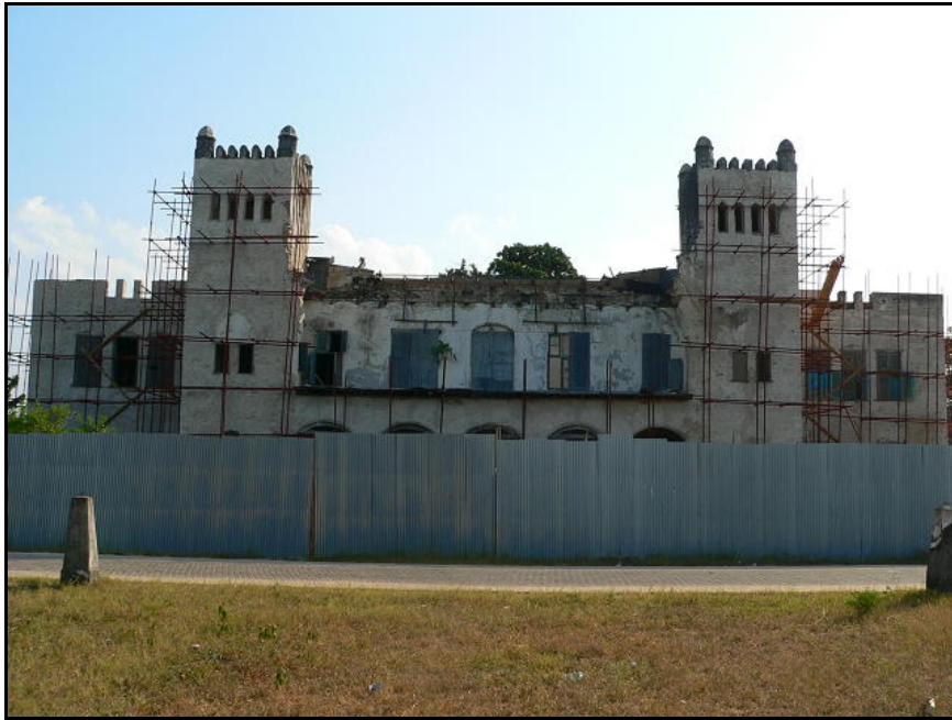
German Boma under Renovation
