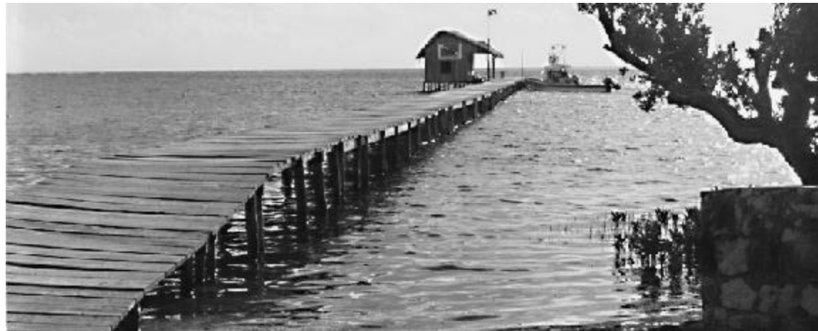
Traditionally, small-scale piers are constructed with wood on pilings.
