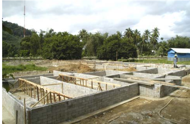
The first level of the Kamphuan Community Learning Center is completed
