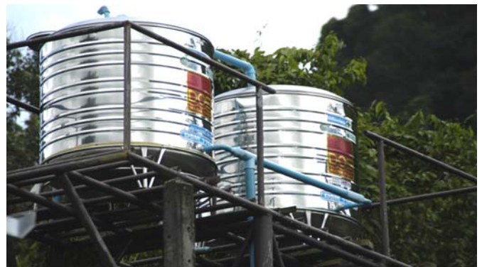
2 1000 liter village water supply system storage tanks were installed at the Ban Talay Nok village water tower
