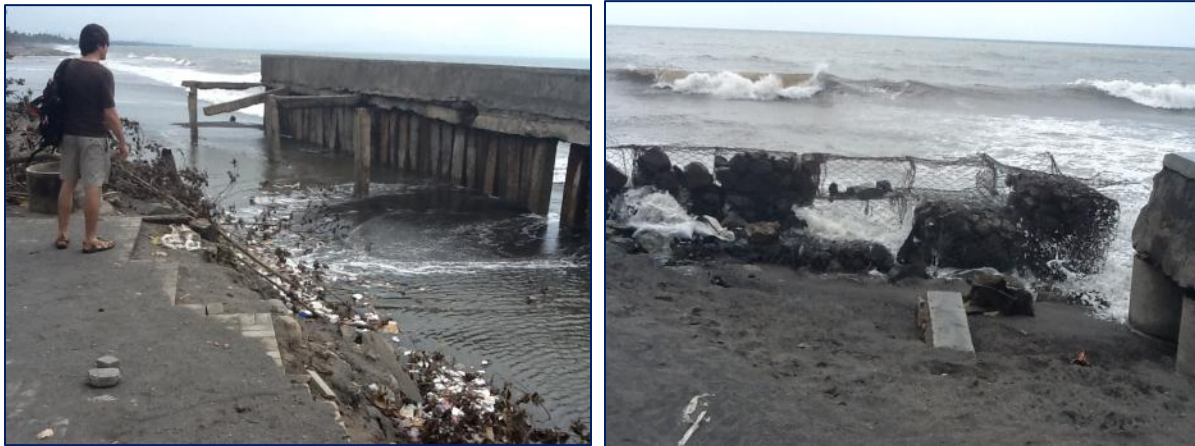
Costly engineering attempts of erosion control that failed in Mataram City
