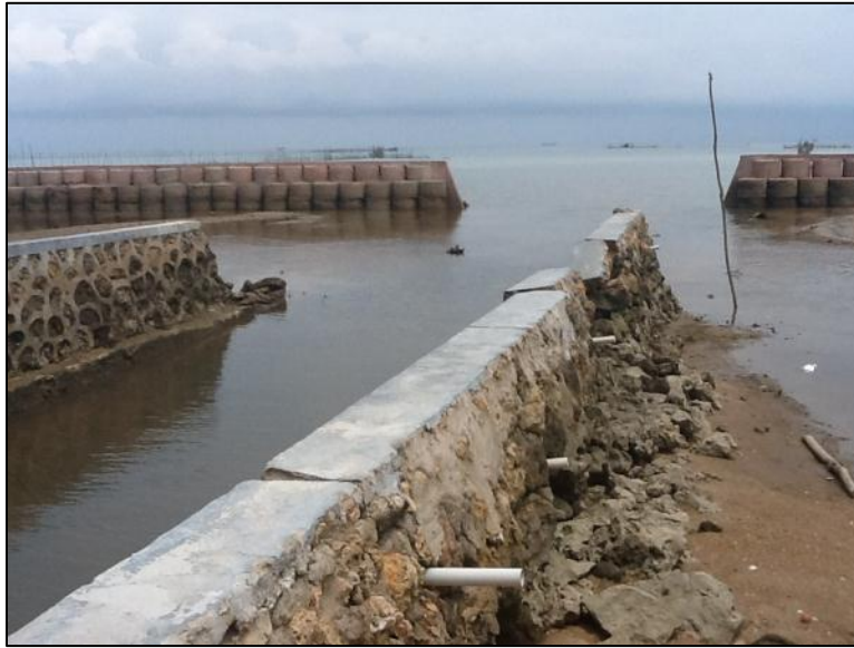
Coastal infrastructure at risk: recent dikes built along a stream bed that drains to the ocean showing storm damage from high waves and subsequent seawall construction further out built to protect the river diking
