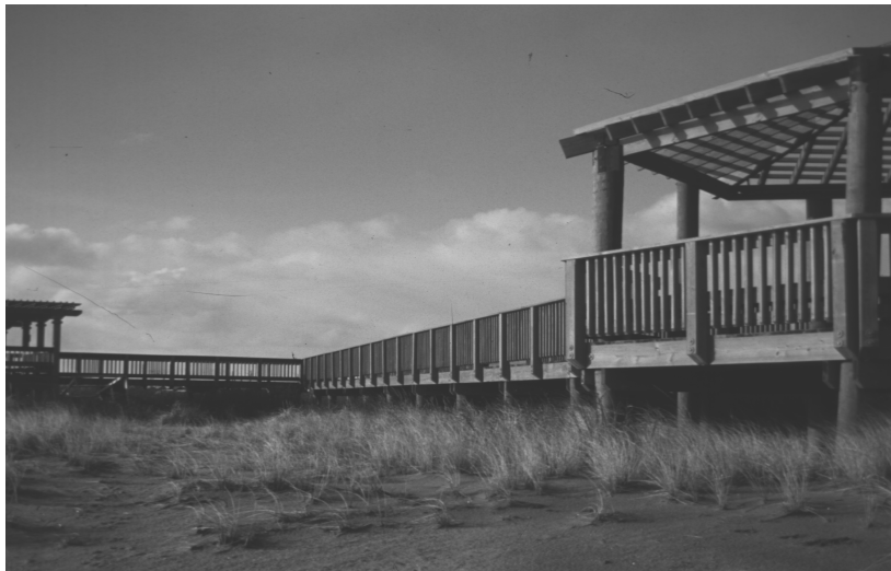
Elevating structures above the height of the vegetation helps maintain vegetation and stabilize the dune.(South Kingston, RI)
