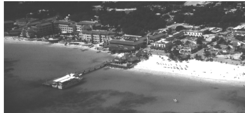
The pier has interrupted the natural flow of sand, thereby enhancing erosion on the down-drift side (left) and accretion on the up-drift side (right).
