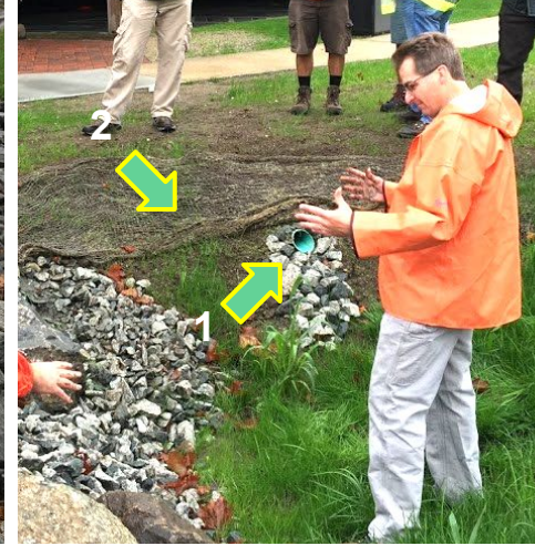
A clear outfall (1) & steep forebay wall (2)
