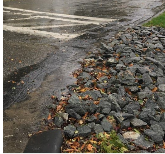
Mounded riprap inhibits water entry
