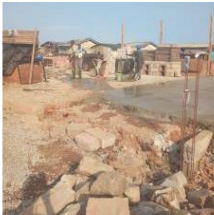
Figure 4 CEWEFIA fisheries training center at Elmina in the Central Region
